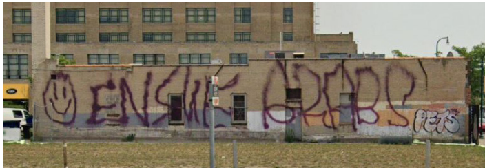
Hamdi Restaurant before Restore-Rebuild-Reimagine Fund support
